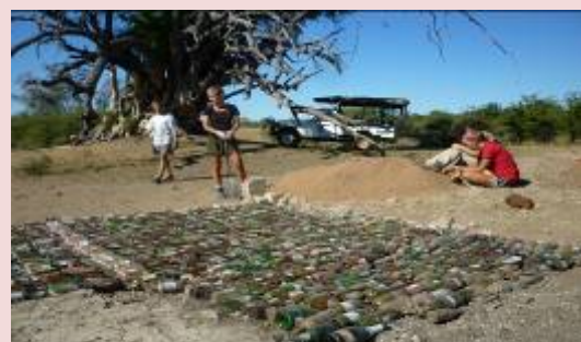
Below: sand filled glass bottles for the tent plinth foundations
